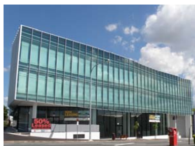
45 Commercial Rd, Newstead completed construction in March 2008. The project was pre-sold by local developers to Opus Funds Management for an end value of $30.4 million. The building contains one level of commercial/retail space and two upper office floors, one of which has been leased.
